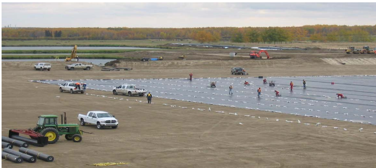
Installation of HDPE Liner
